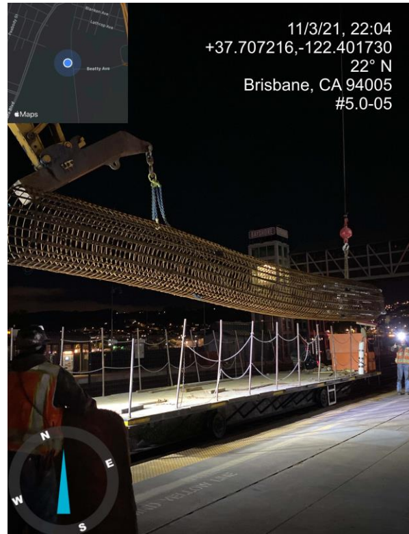
Preparing to Set Rebar Cage in Segment 1B
