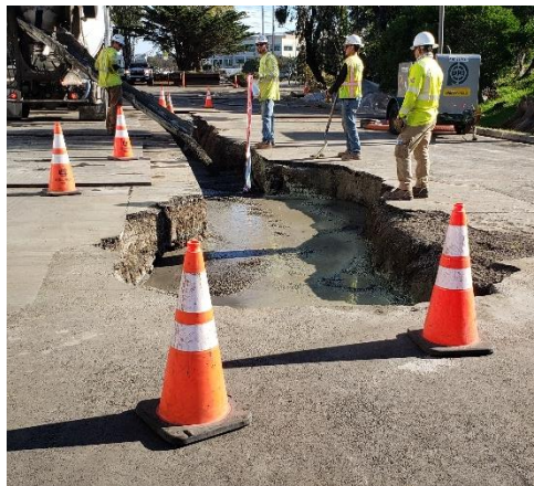
Backfilling Circuit #2 ductbank with slurry in the HealthPeak parking lot
