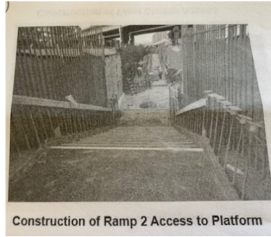
Ramp under Construction
