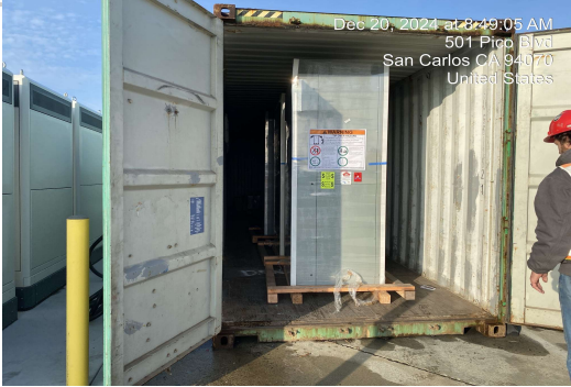
switchboard MDPO-2 was delivered to south base
