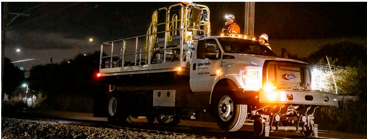
Balfour Beatty Night Wire Work
