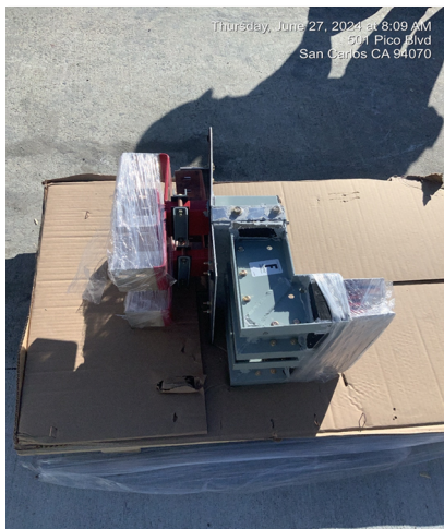
The Bus Duct Issue: the cellophane-wrapped part (left photo) of the bus duct does not connect into the MDPO-1 switchgear (right photo). The Resident Engineer and Anvil Builders are researching solutions.
