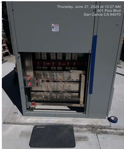
The Bus Duct Issue: the cellophane-wrapped part (left photo) of the bus duct does not connect into the MDPO-1 switchgear (right photo). The Resident Engineer and Anvil Builders are researching solutions.
