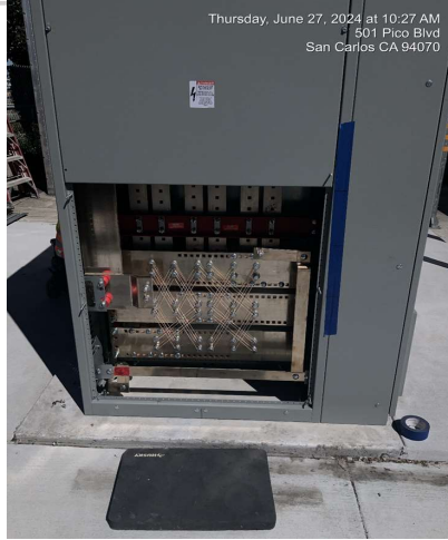
The Bus Duct Issue: the cellophane-wrapped part (left photo) of the bus duct does into connect into the MDPO-1 switchgear (right photo). The Resident Engineer and Anvil Builders are researching solutions.
