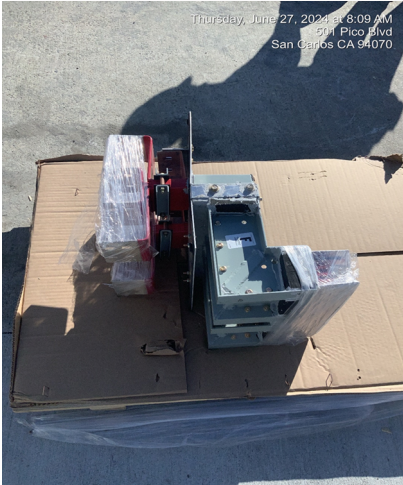
The Bus Duct Issue: the cellophane-wrapped part (left photo) of the bus duct does into connect into the MDPO-1 switchgear (right photo). The Resident Engineer and Anvil Builders are researching solutions.
