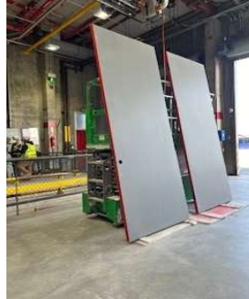
Central Doors are ready to install
