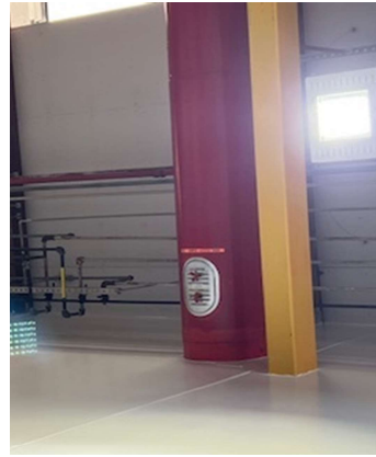
Fire Damper Door installed (NB Building 100)
