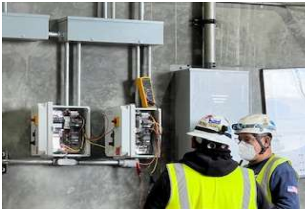
Gas Detection system testing (NB Building 100)
