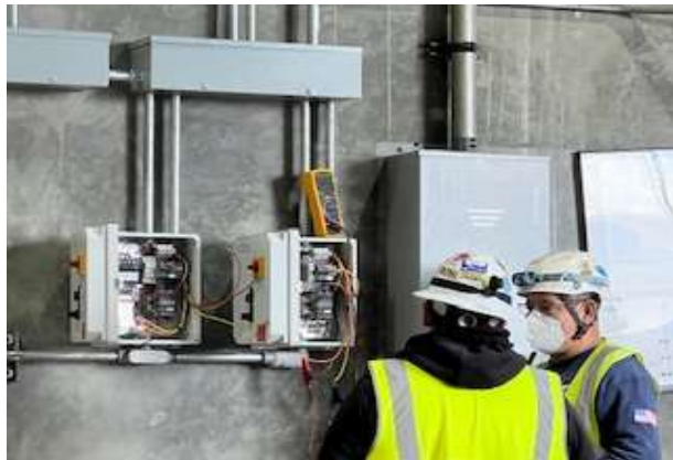
Gas Detection system testing (NB Building 100)
