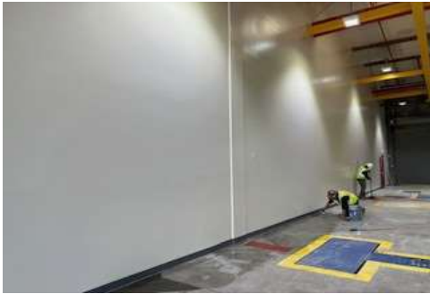
Cleaning commenced. (NB Building 100)
