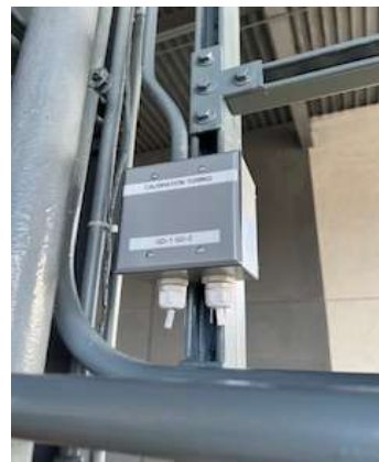
Building 500 – Gas Detection System installed and tested
