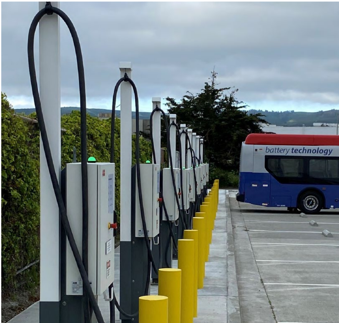
Figure 5-6. North Base - Interim BEB Chargers
