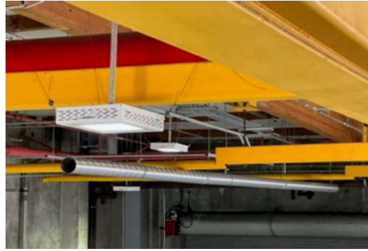
All lighting - lowered 24" from the ceiling
