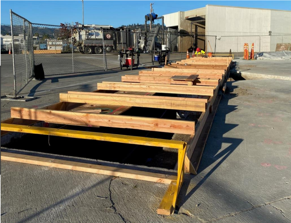
Construction of Charger Pads.
