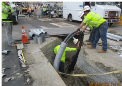
Routing from splice box to termination point
