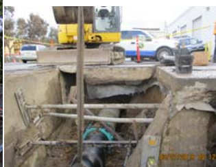
Water main tie in East Grand Ave.
