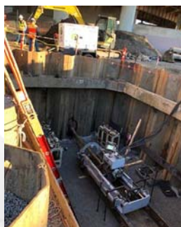
Shoring and Main installation - West Plaza
