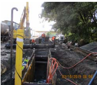
18 inch water main East side UPRR track
