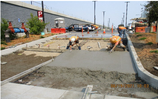
Photo 3 - New Driveway for Bike Path
