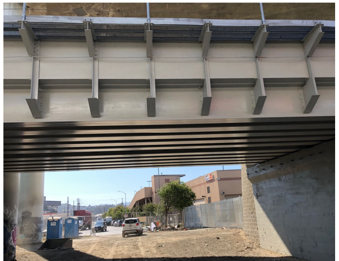
Photo 4 - New Napoleon Bridge
