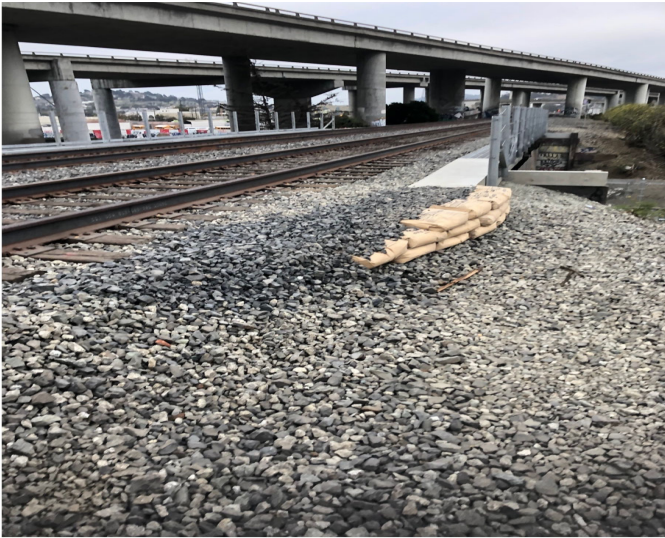
Photo 1 - Marin Street New Walkways
