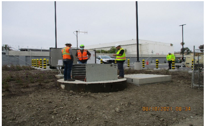
Photo 2 - Pump Station Testing
