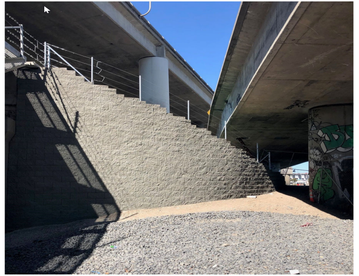
Photo 2 - Napoleon Northeast Retaining Wall
