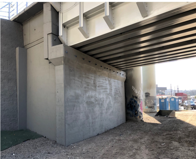
Photo 3 - Napoleon South Abutment
